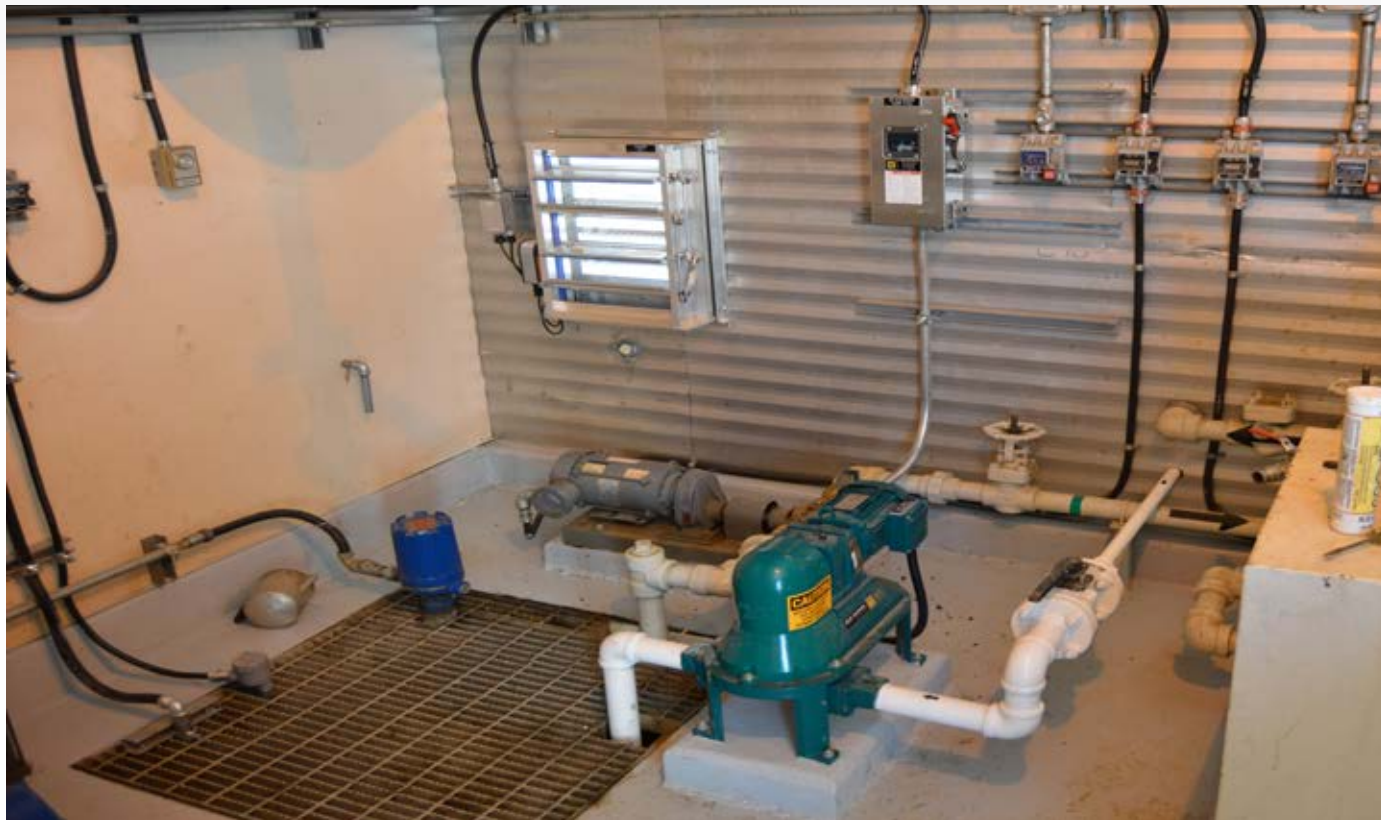
Mud Sucker 2FAC-EC installed at a wastewater pump house. Sump application. Pump transfers up to 20 GPM of wastewater and light solids. Shown with a three phase Siemens electric motor and SEW Eurodrive gear box. Other drive systems available.
