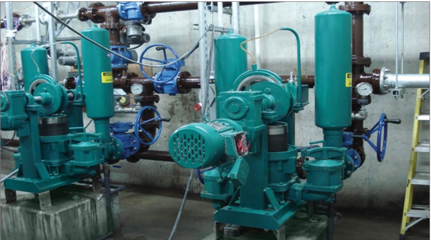
This Space Saver in Washington State replaced an existing double disc pump installation. No piping changes were needed because the pump configuration is similar.
