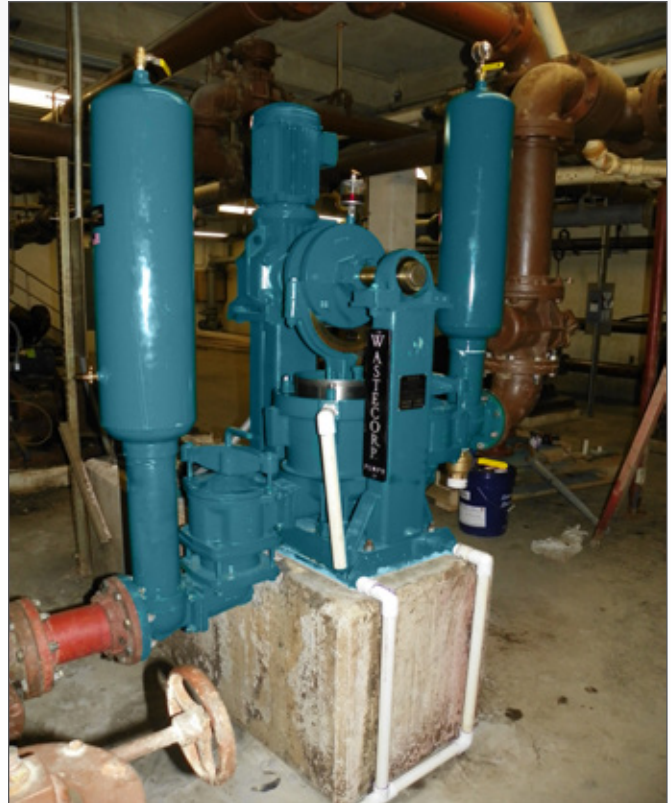
Wastecorp PE-741 SS Series shown at a meat packing facility. Pump shown with optional piped in stuffing box and pump base in white pvc (additional colors and materials available).
