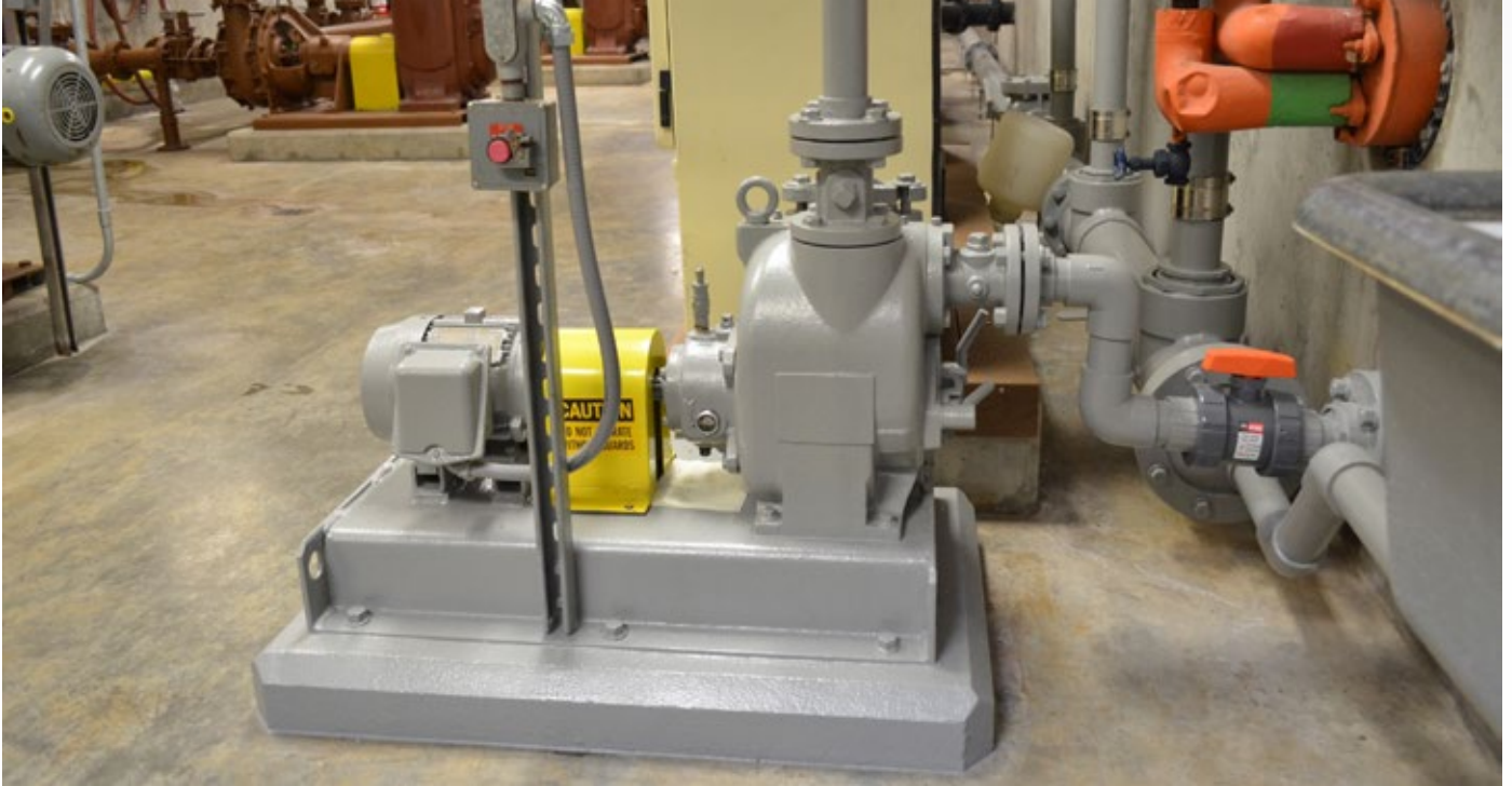
WASTEWATER PUMPS Shown: Trash Flow TFCC-2 installed at a Connecticut wastewater treatment plant. Direct drive model shown. 2" connection with pumping capabilities up to 210 GPM.
